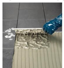
then a white adhesive should be used to prevent any shadowing through the stone and grout from the adhesive below. Mix the adhesive as per the instructions by adding the powder to clean water and stir until a smooth, lump free consistency is obtained. Mix only enough adhesive which can be used within the pot life of the product (approx. 30 minutes at 20°C).
