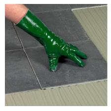
Using a suitable, solid-bed notched floor trowel held at a 45° angle, spread the adhesive onto the floor to form parallel ribs into which the tiles should be pushed with a firm twisting action, this will collapse the ribs of adhesive and produce a 3-4mm solid bed of adhesive beneath the tiles. Work in small areas and discard any adhesive that begins to dry or 'skin over'. Tiles with deeply keyed back
