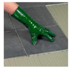
Remove deposits of adhesive which may build up in the gaps between the tiles. DO NOT WALK ON THE TILES UNTIL THE ADHESIVE HAS SET, this is generally 3 hours approx. for rapid setting adhesives or 24 hours approx. for standard set adhesives.
